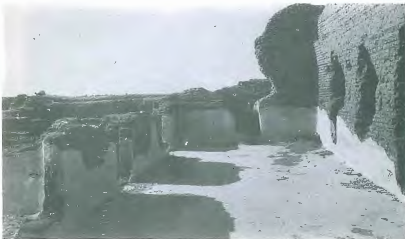
b The eastern corridor of the new residential building
