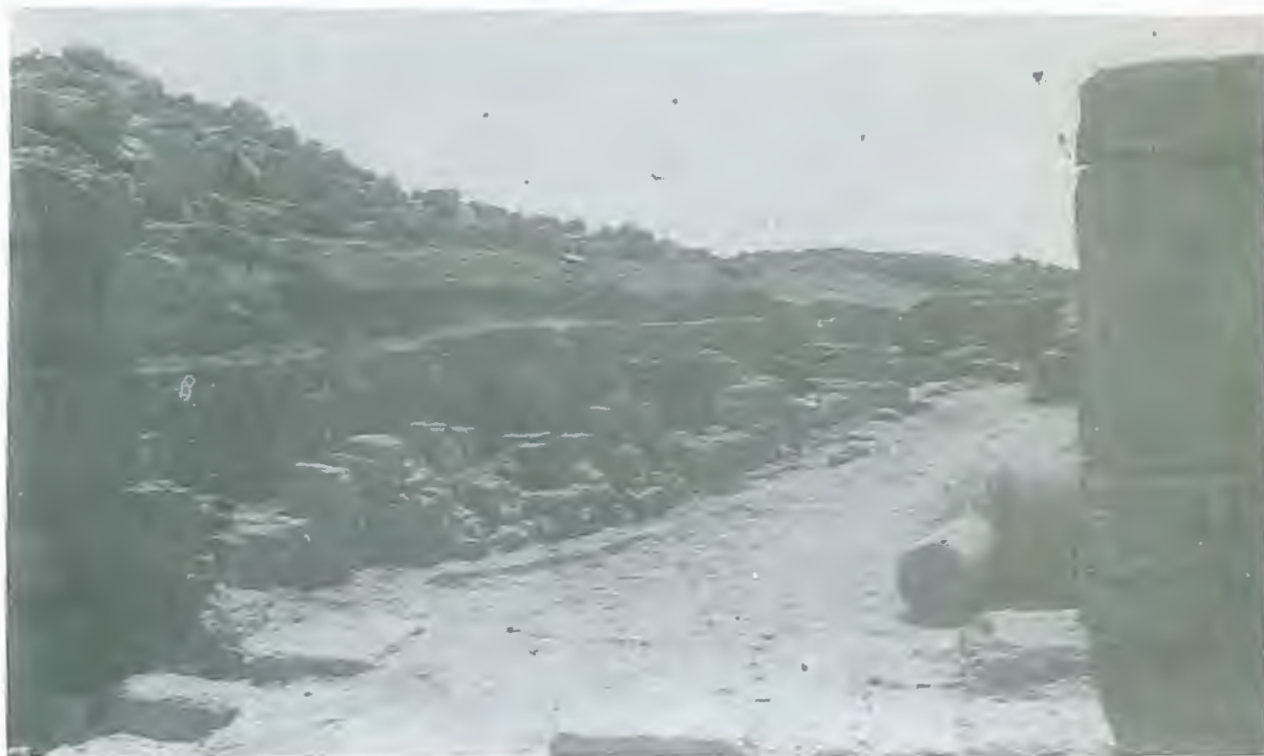
a. View from the pilgrimage court to the new western street
